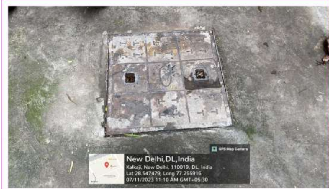
Rain Water Harvesting Pit
